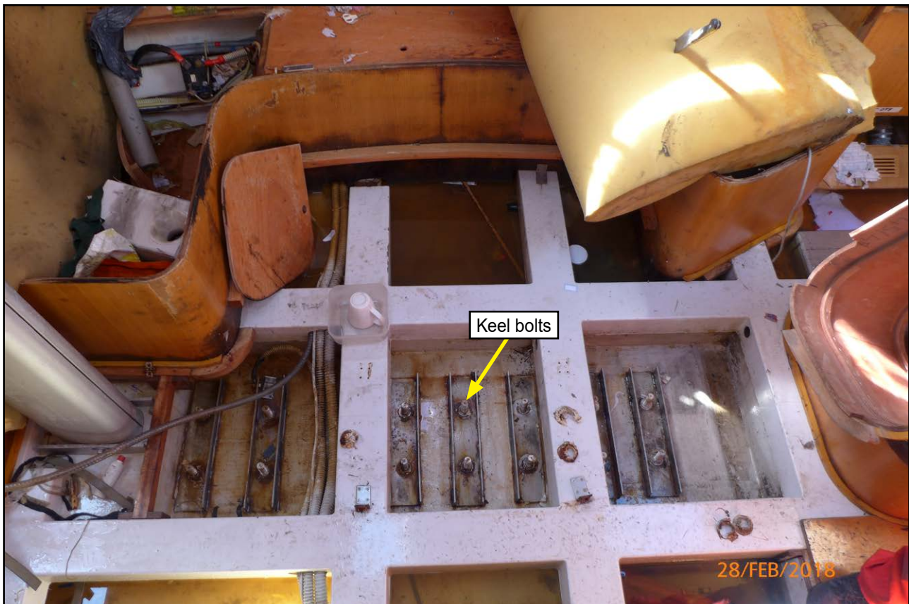
Figure 13: The keel matrix (bolts removed by surveyor prior to keel plate removal)
