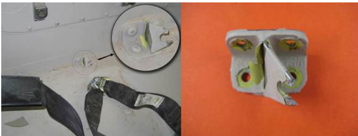
Figure 16. Location of harness attachment and close-up of fracture
